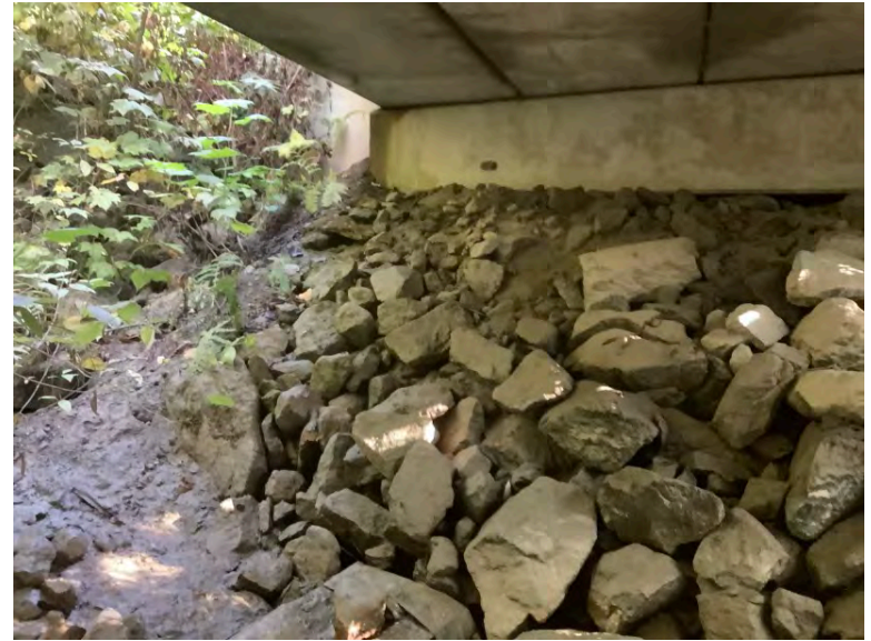
Left Bank Abutment when facing downstream
