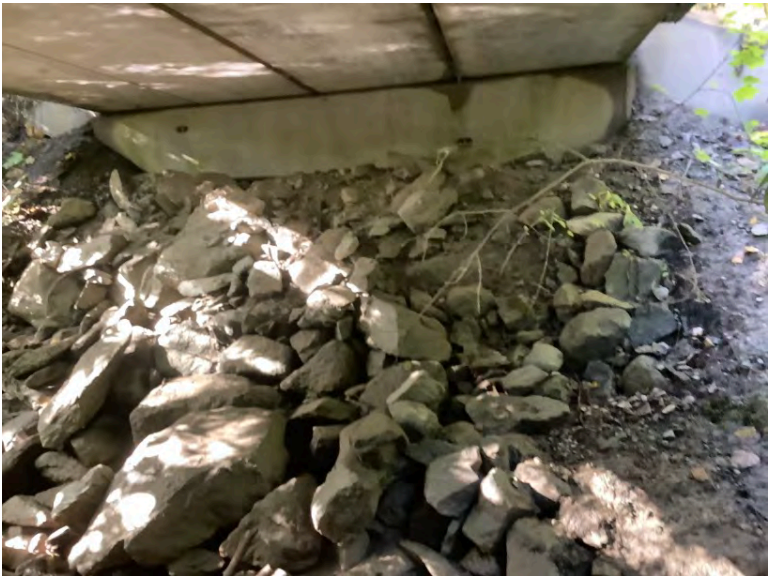
Right Bank Abutment when facing downstream
